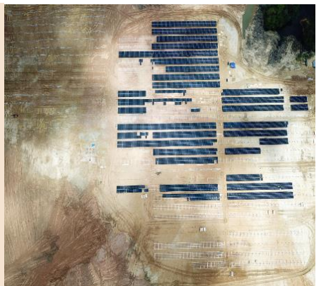
Progress of solar panel installation at Tarjun Plant, South Kalimantan (Feb 2024)
